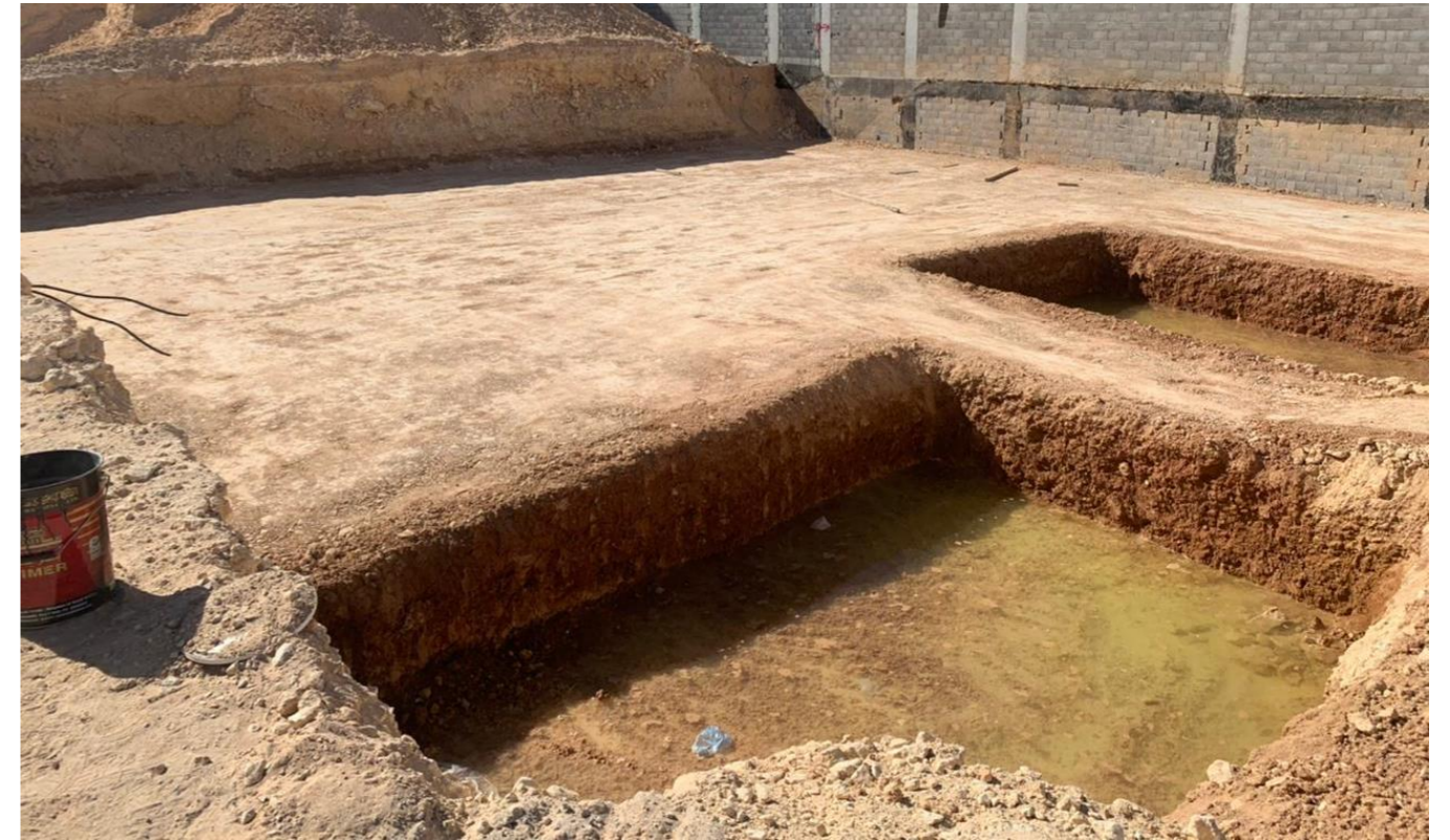
Excavation work and reach the base to the level of establishment
