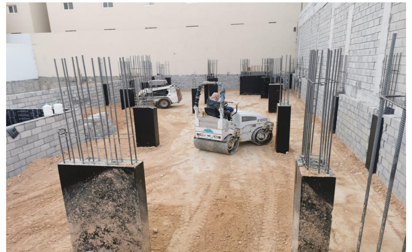
Cover the pad foundation, as well to the columns
