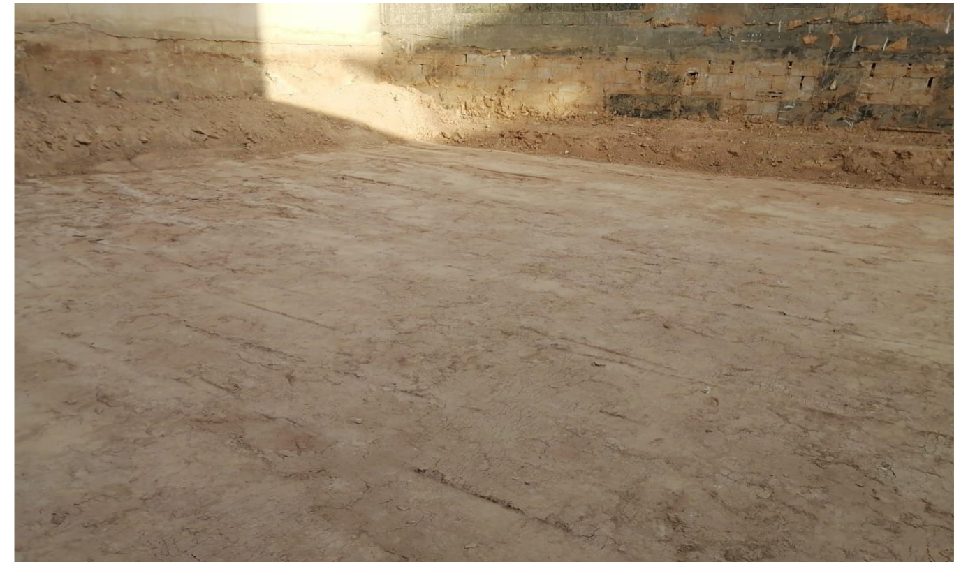
Photos illustrating the quality of work on the site
