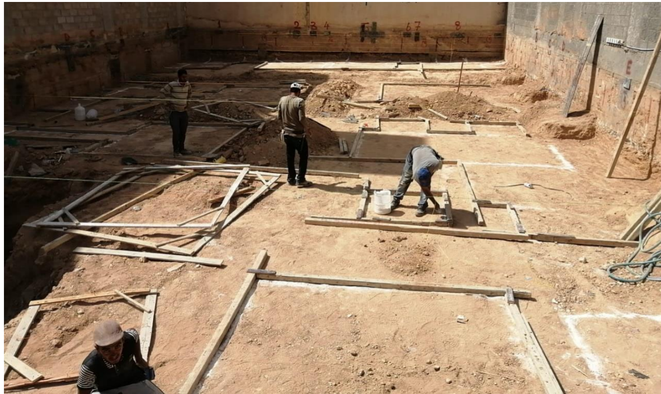
Photos illustrating the quality of work on the site
