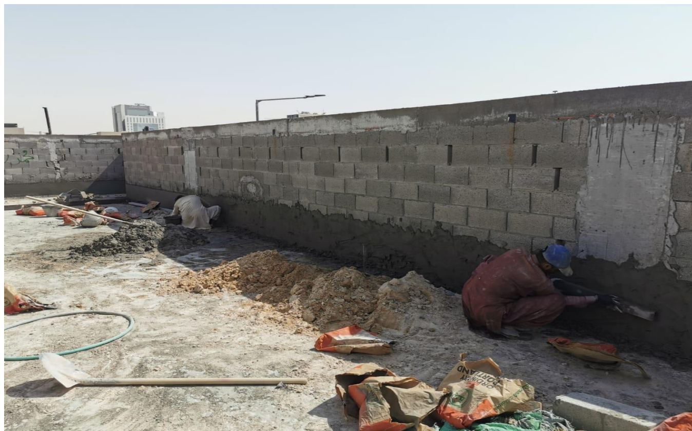
Plaster works with wall isolation
