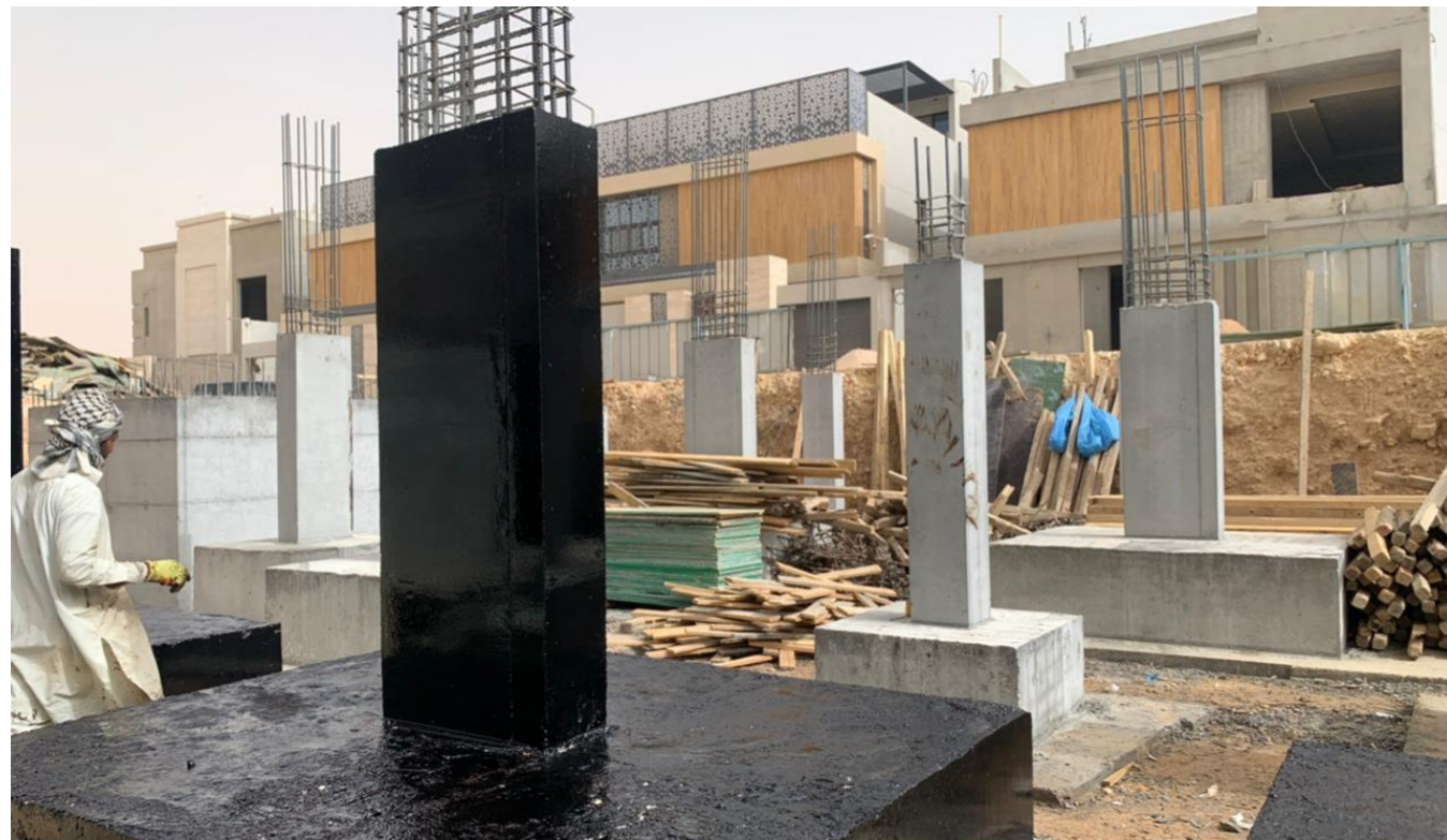
Pad foundation moisture insulation works, column and wastewater
