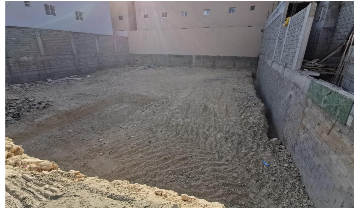
Raising land levels, leveling heights and dropping base locations topographically
