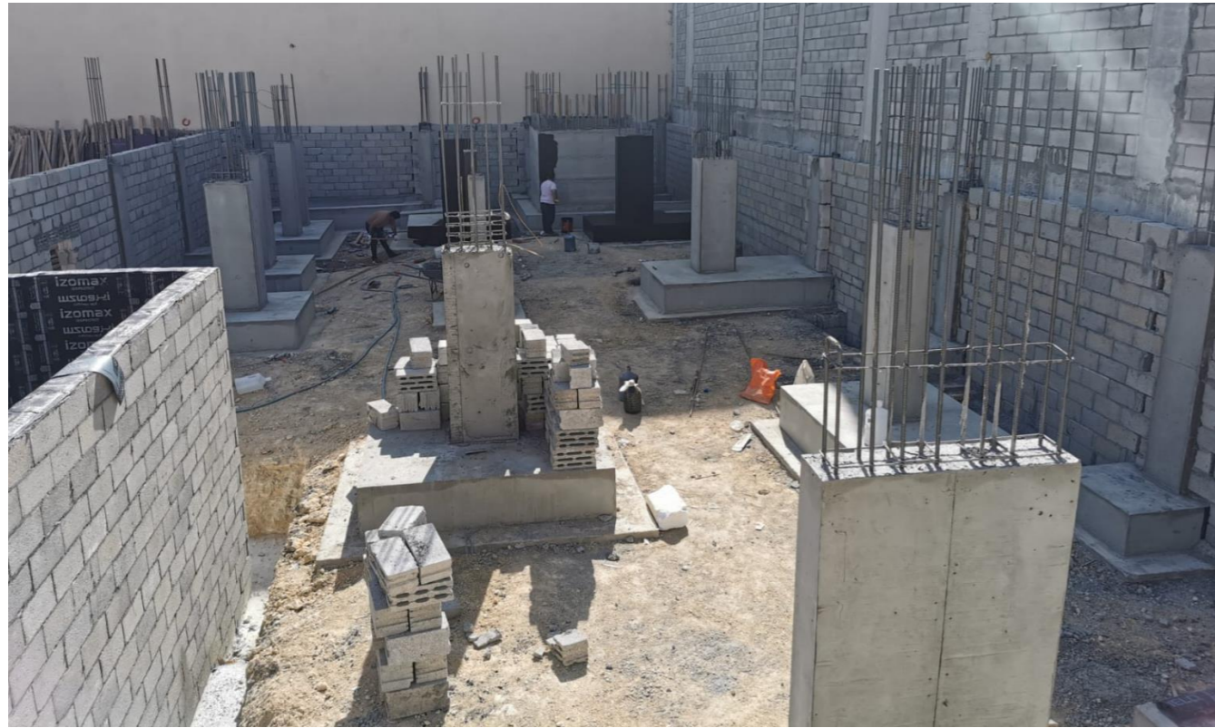
Cleaning casting works, dropping pad foundation points and carpentry works
