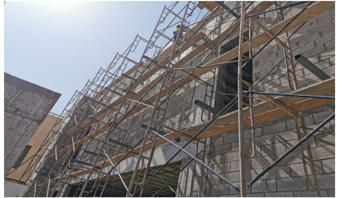
Installation of the bases of the front décor
