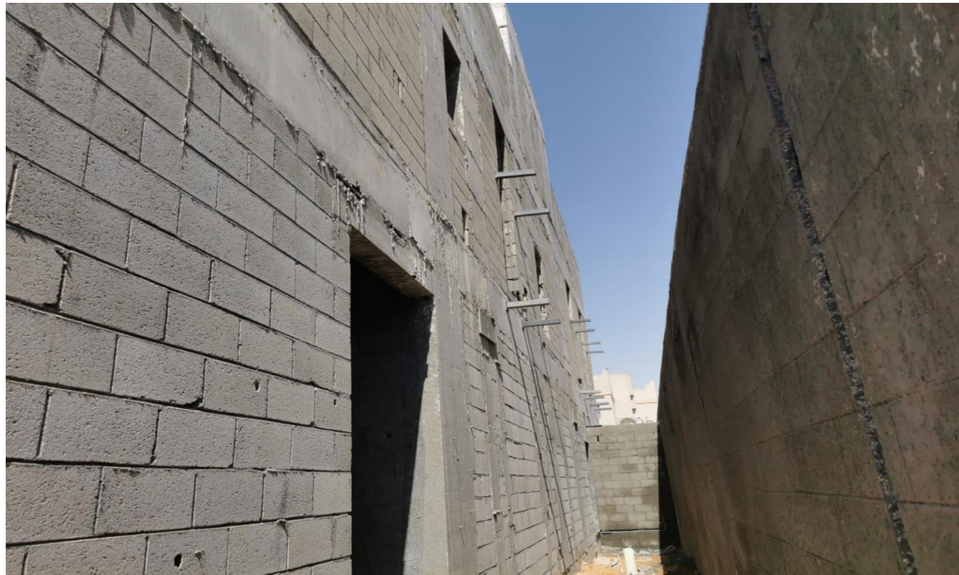
Installation of bases of the eastern windows
