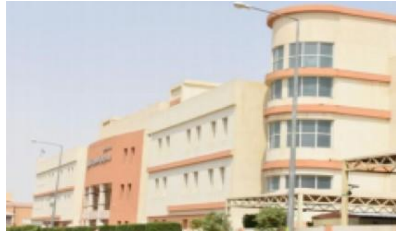
otos from the project of Al-Jawdah schools complex in Riyadh
