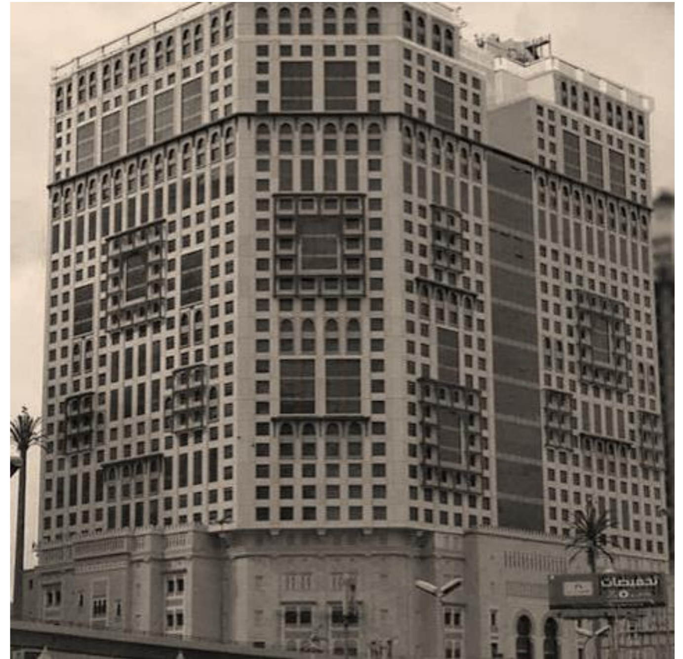
Preparation of contractual studies and expertise for “Anjum Hotel” project Near to the Holy Mosque MASJED ALHARAM Mecca.
