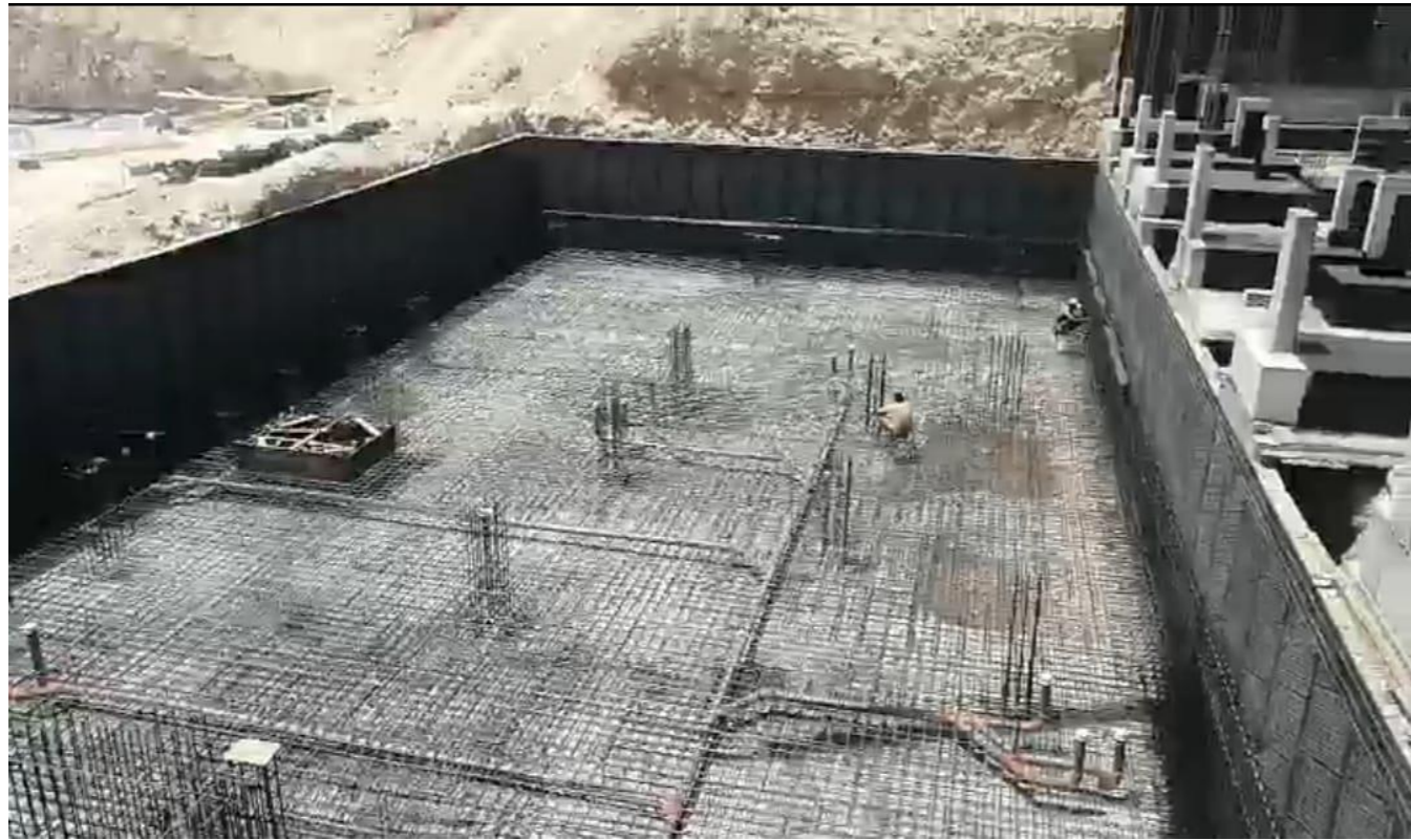
Blacksmithing, carpentry and pour concrete to the basement columns
