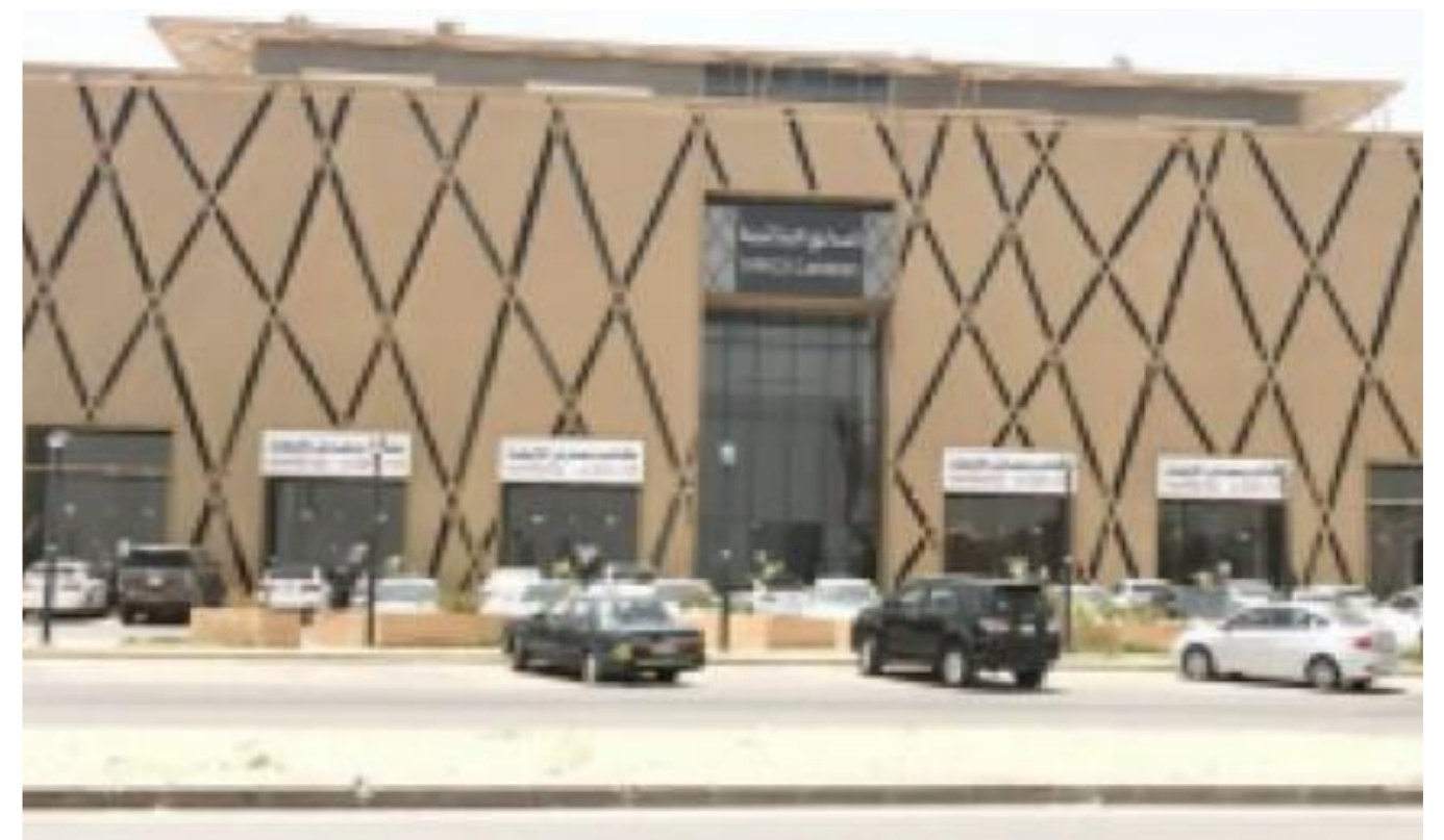
Technical supervision of a number of commercial and residential buildings in the city of Riyadh
