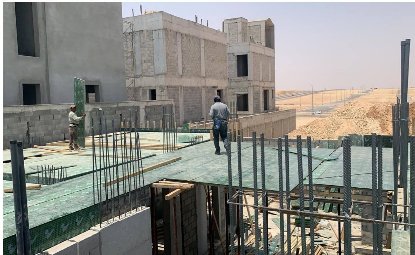
Carpentry, blacksmithing and casting of the ground roof floor and stairs
