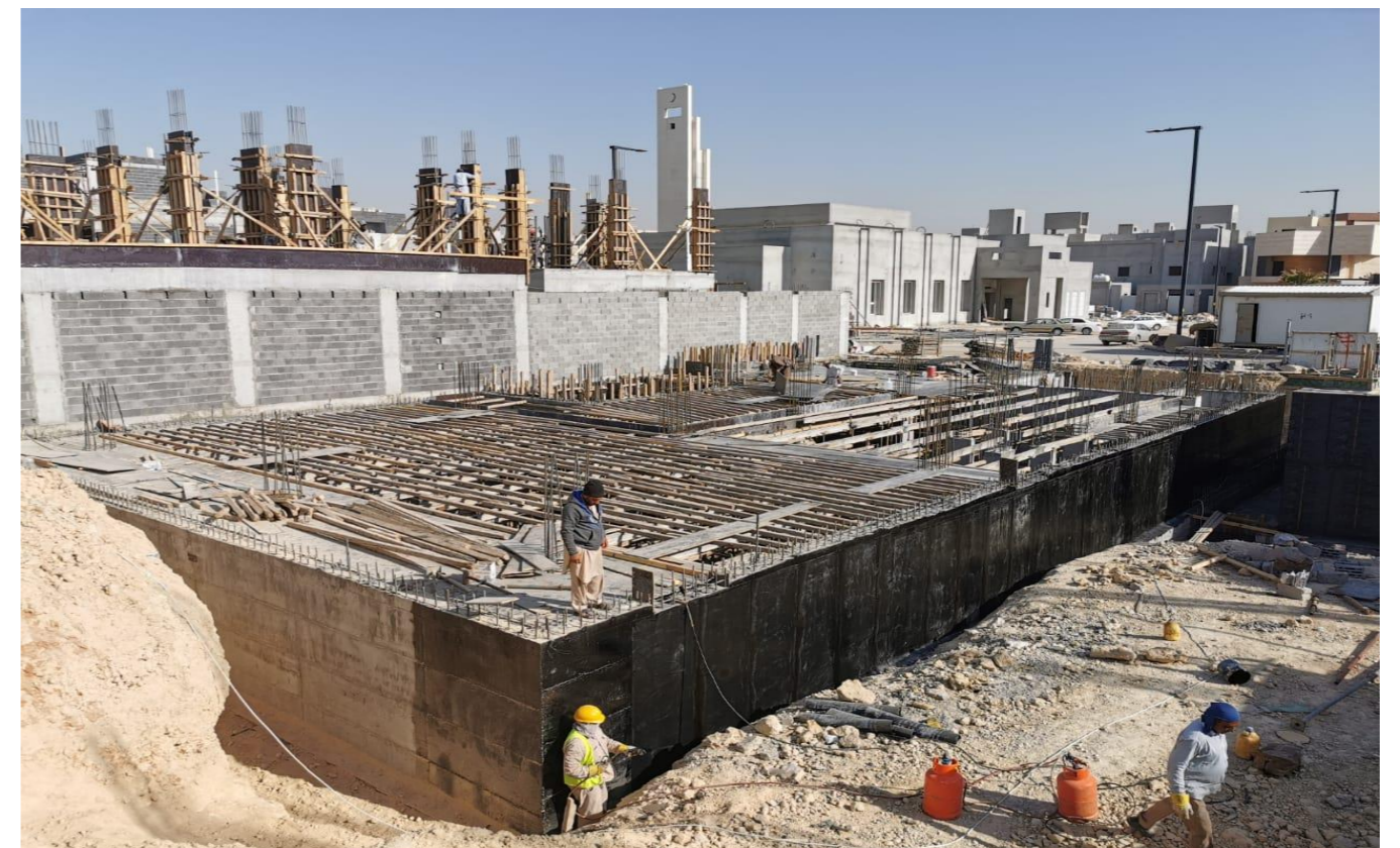
Carpentry, blacksmithing and pour concrete to the basement floor's roof
