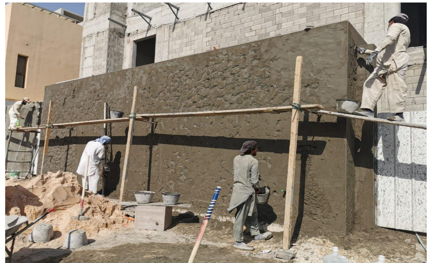
Exterior wall plaster
