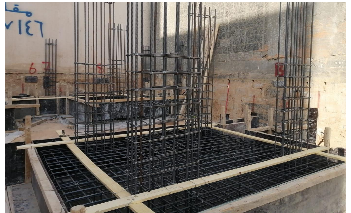
Burial works around the bases and column necks
